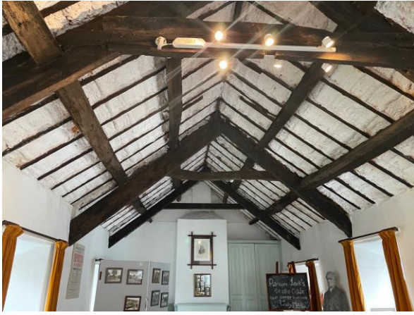
Internal Roof Space
