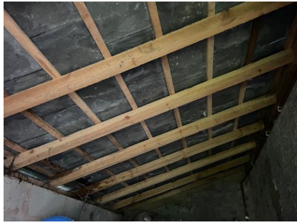
Internal Roof Felt and Batten
